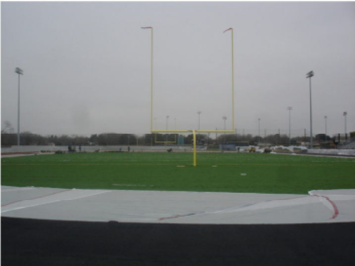
L. D. Bell High School – Overall view of field turf progress.
