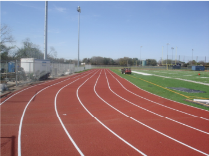
L. D. Bell High School – Completed lane striping.
