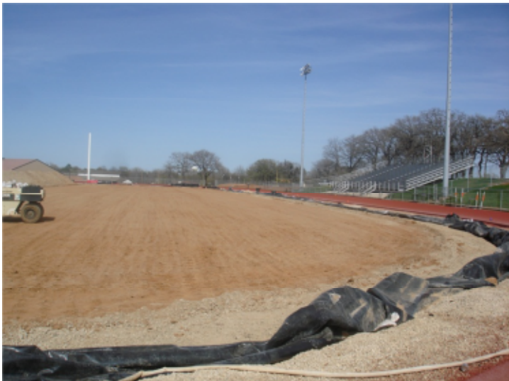
Trinity High School – Subgrade work of field.
